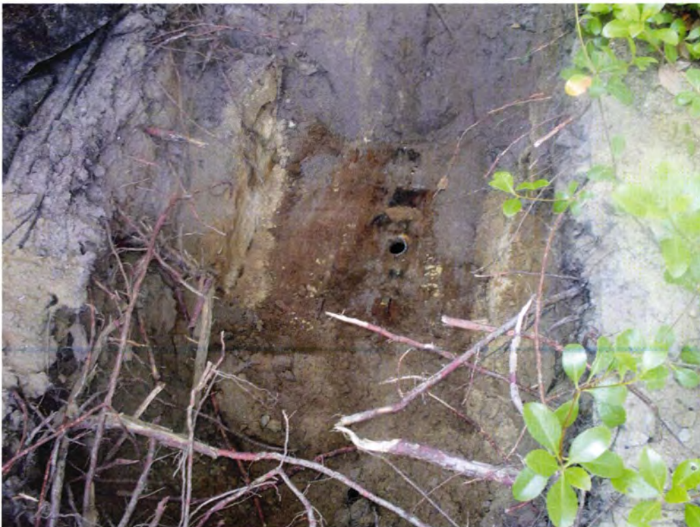
Picture 2: UST 341Ash excavation in progress.
